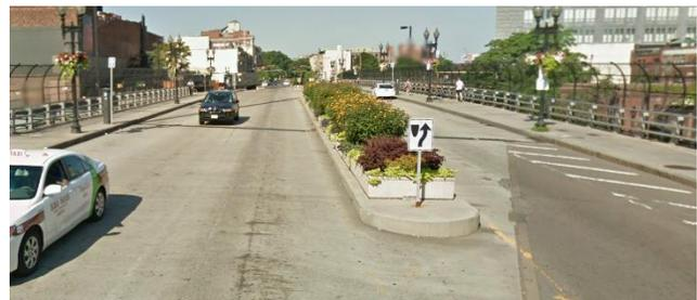
eliminates mid-block crossings. While a fence can encourage higher vehicle speeds and is unacceptable to the community, planters add value to the community and slow traffic. If the vertical split of the north and south sides of the overpass presents a problem, narrower planters can be installed separately on the two sides.
